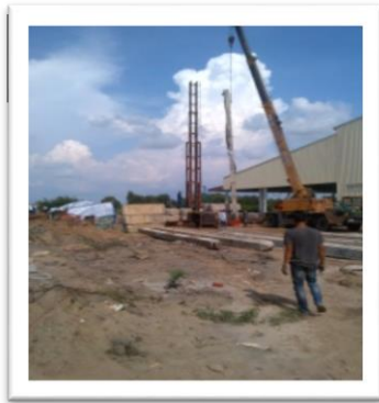
Đóng cừ Timber Pile Driving
