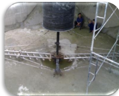
Dàn cào bùn Clarifier scrapper fabrication & installation
